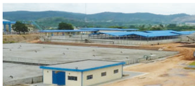
Figure 1: Location map of Lower Usuma Dam treatment plant
