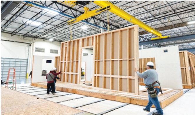
Figure 2: Factory settings of modular construction (vbc.co)
