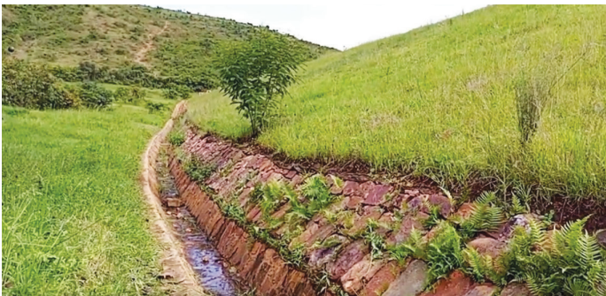
Figure 15: Sample photo of slope toe with erosion control structures (Source: https://www.youtube.com/watch?v=GS0aL9FX0vo )
