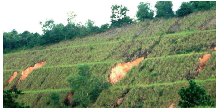
Figure 6: Localised Erosion on Slope (Gue & Tan 2003)
