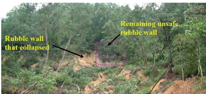
Figure 11: Collapsed rubble wall at Taman Hillview failure site (Gue & Tan 2006)
