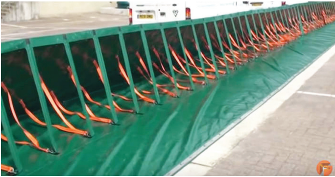
Figure 6: The Rapidam Mobile Flood Wall Barrier (Chandra Mouli et al. , 2018)
