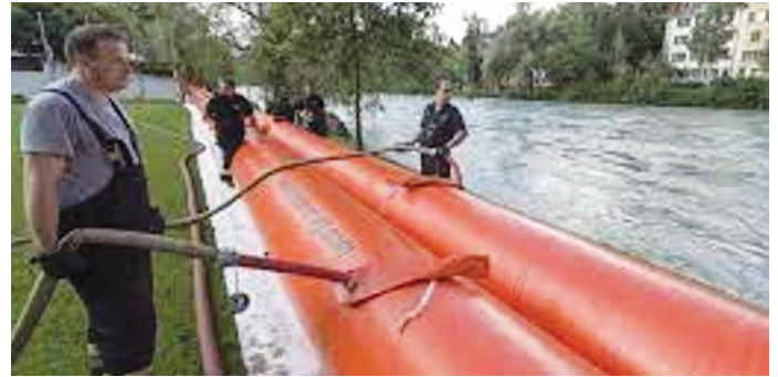
Figure 7: The Beaver® Storm and Flood Protection System Mobile Flood Wall Barrier (Beaver® Protection Systems, 2019)
